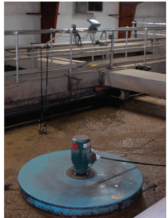
Figure 1: Anoxic Zone with floating mixer (TriOxmatic®, VARION® and SensoLyt® Sensors in background)
